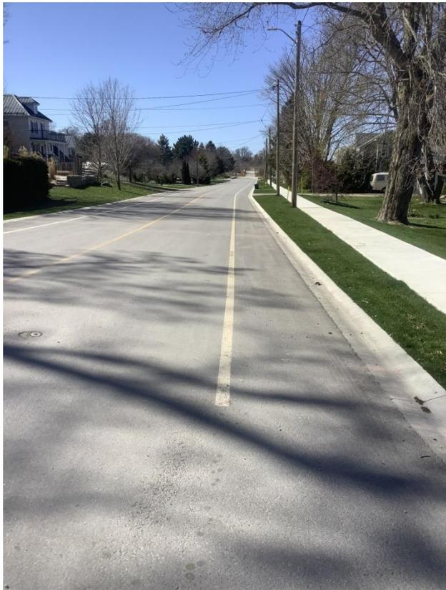
Proposed Peel St travel width requirements 10.2 metres – 3.75 metre vehicle, barrier curbs, 2.7 metre MUT = 10.2 metres. Slightly more room for tree retention
