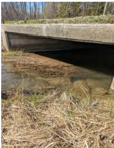
PHOTO 9: Large box culvert southwest side of Highway 26
