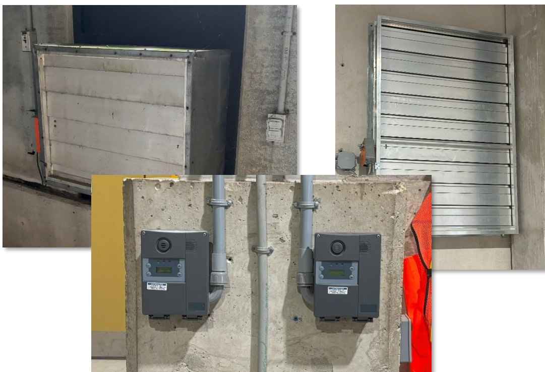
Figure 2.2 Craigleith WWTP New Exhaust Air Louver Controls
