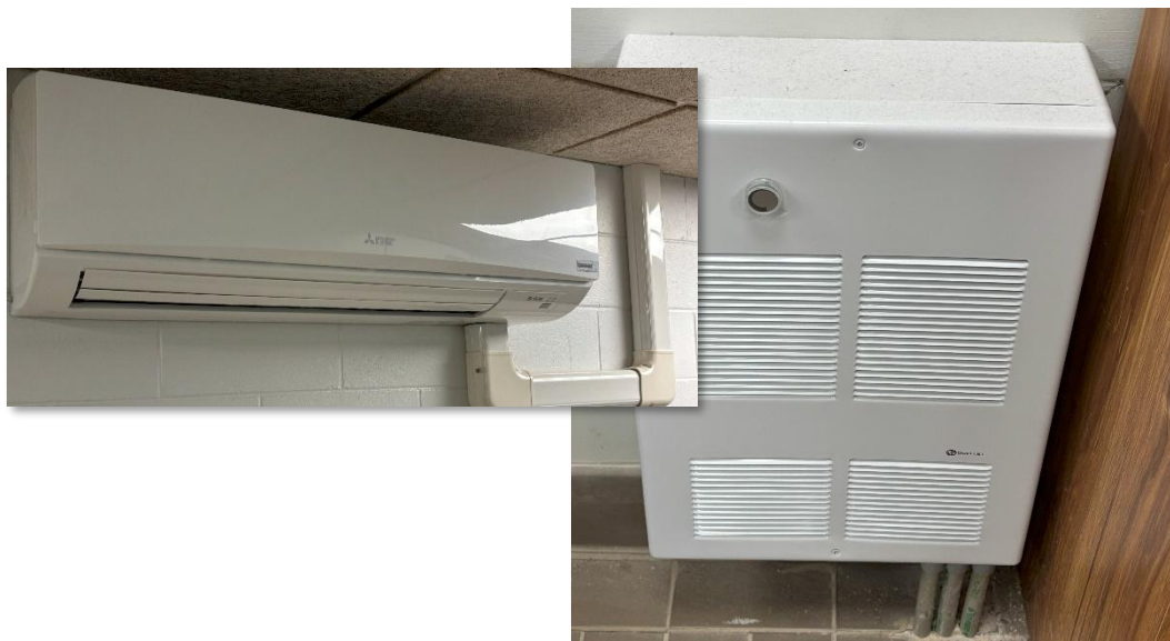
Figure 2.1 Craigleith WWTP Air Source Heat Pump and Unit Heater Upgrades
