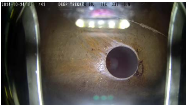
View up into one of two roof vents
