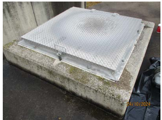
Roof hatch secured and locked after inspection
