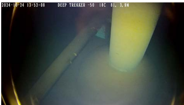
View lower portion of centre roof support pillar
