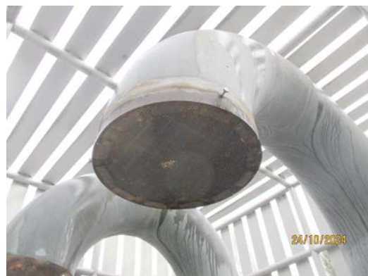
Underside of 2 nd gooseneck vent screen – ok
