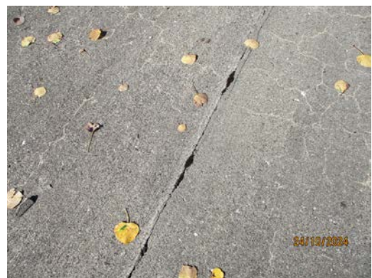
Area of the intersection of topside roof joints
