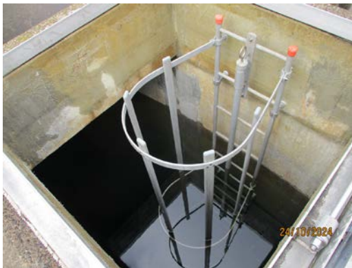
Upper ladder cage and tie off post
