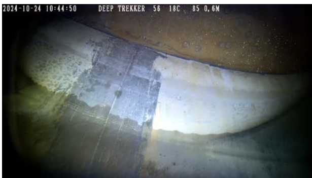
View up at roof to wall joint interface
