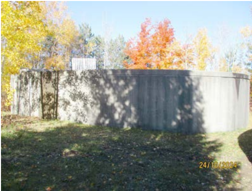
Overall view of the North Reservoir
