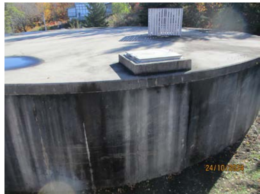
South Reservoir - view from North Reservoir roof
