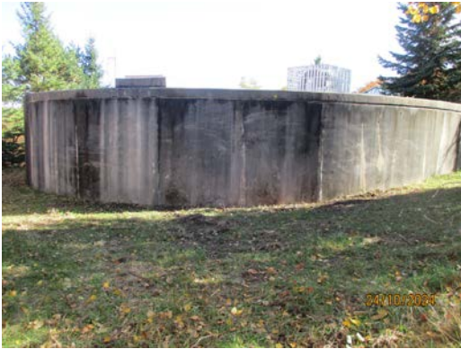
Overall view of South Reservoir
