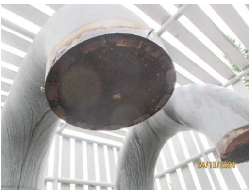
Underside of 1 st gooseneck vent screen – ok
