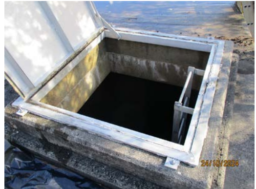
Roof hatch open during video inspection
