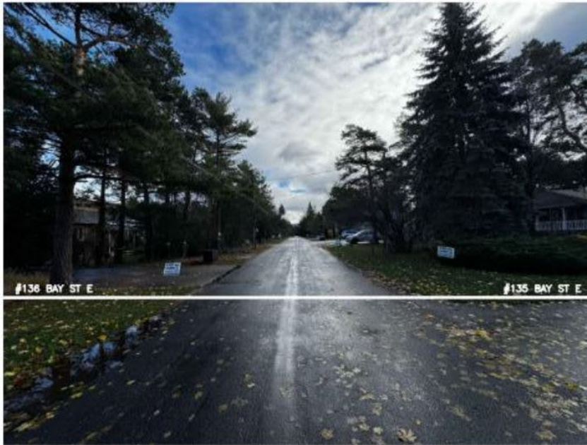
EXISTING CONDITION – 135/136 BAY ST. E.
