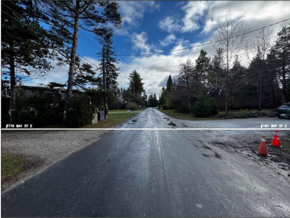
EXISTING CONDITION – 176/181 BAY ST. E.
