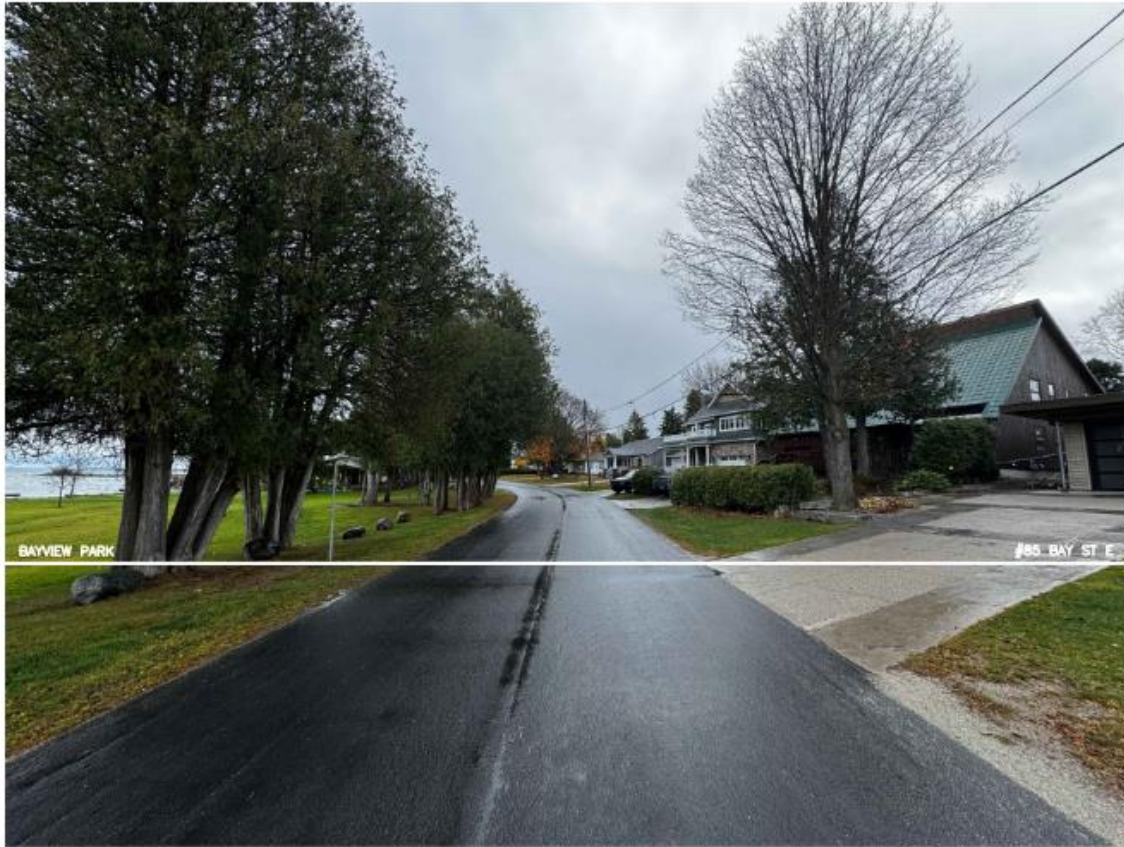
EXISTING CONDITION – 85 BAY ST. E.
