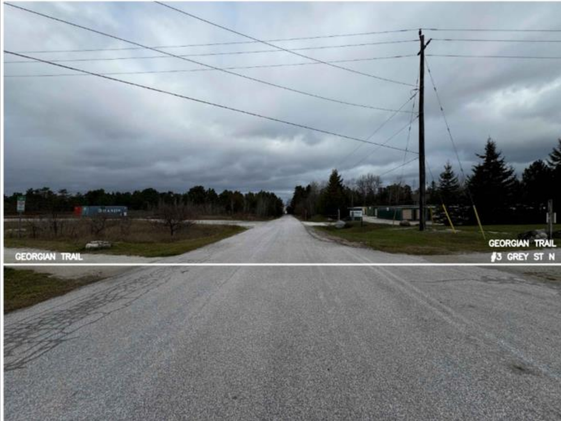
EXISTING CONDITION – GREY ST.
