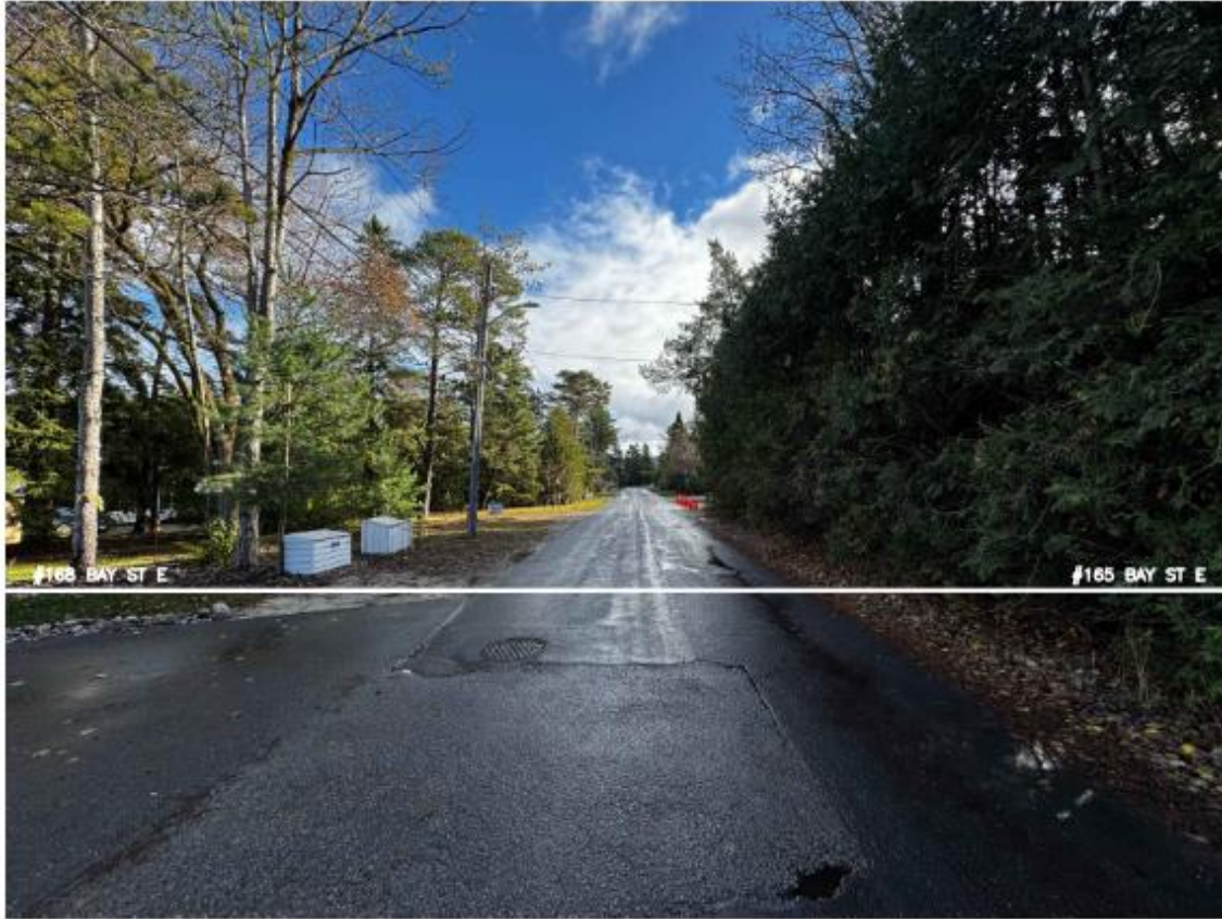
EXISTING CONDITION – 165/168 BAY ST. E.
