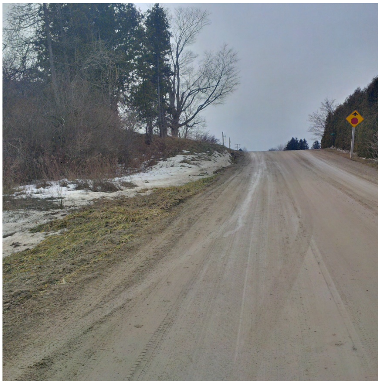
Pic 2 - Peel Street at King Street Road Allowance
