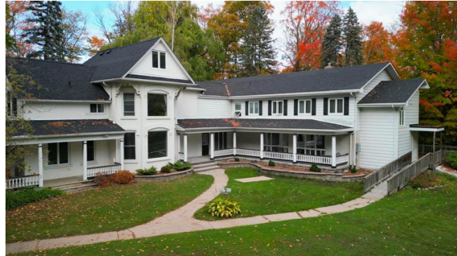
Figure 2. Photo of Existing Building
