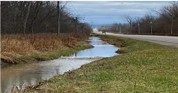
You can see how this LID works to slow down floodwaters from the escarpment and remove turbidity!
