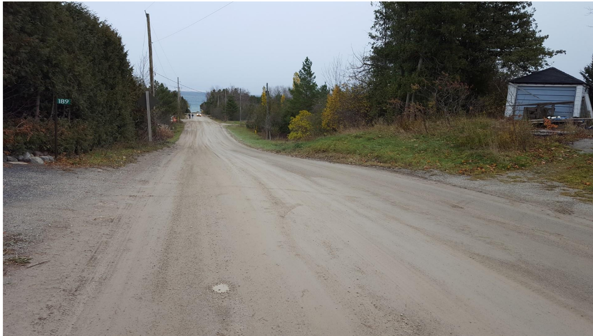
Peel Street North Road Reconstruction
