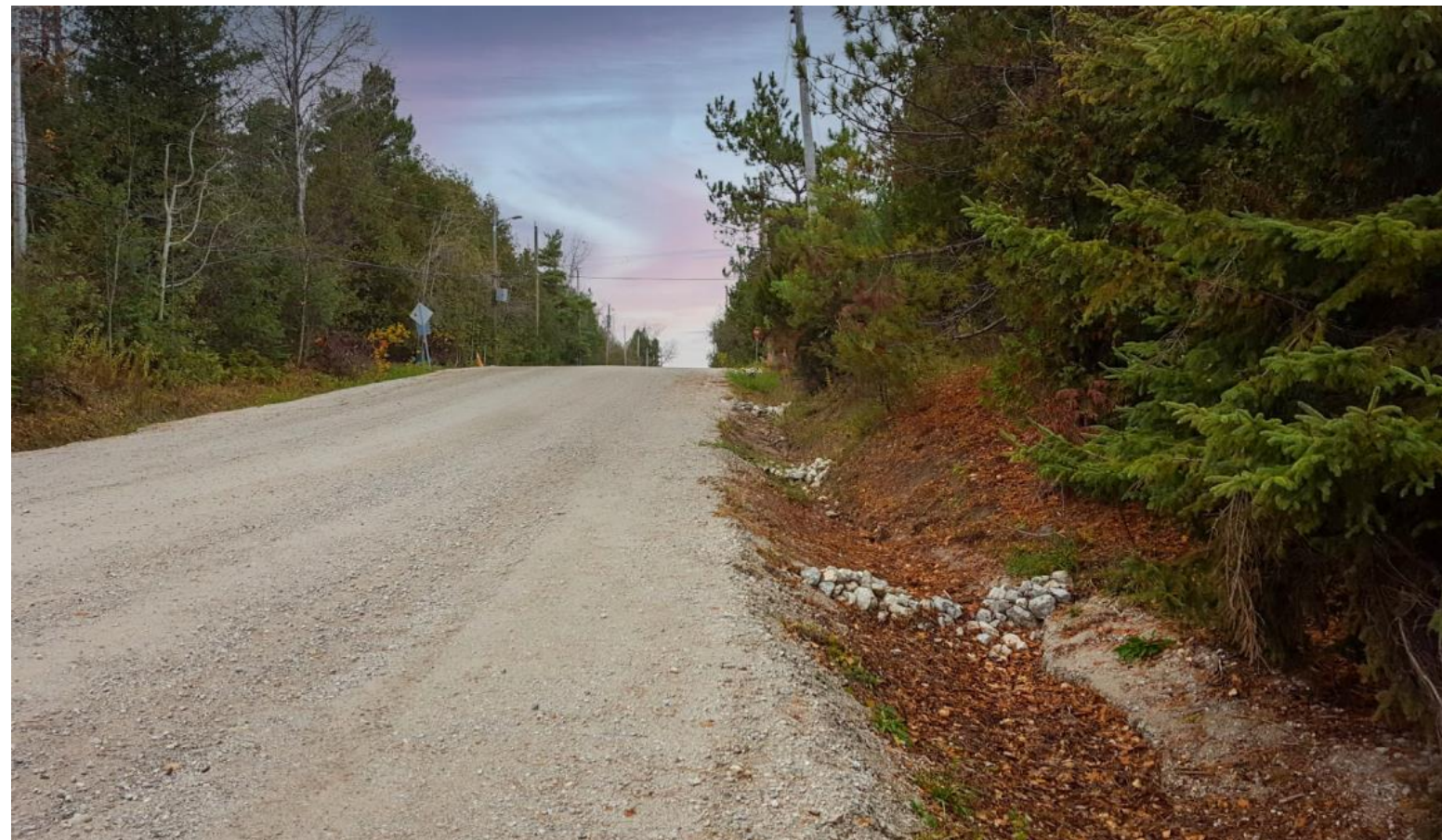
Peel Street North Road Reconstruction
