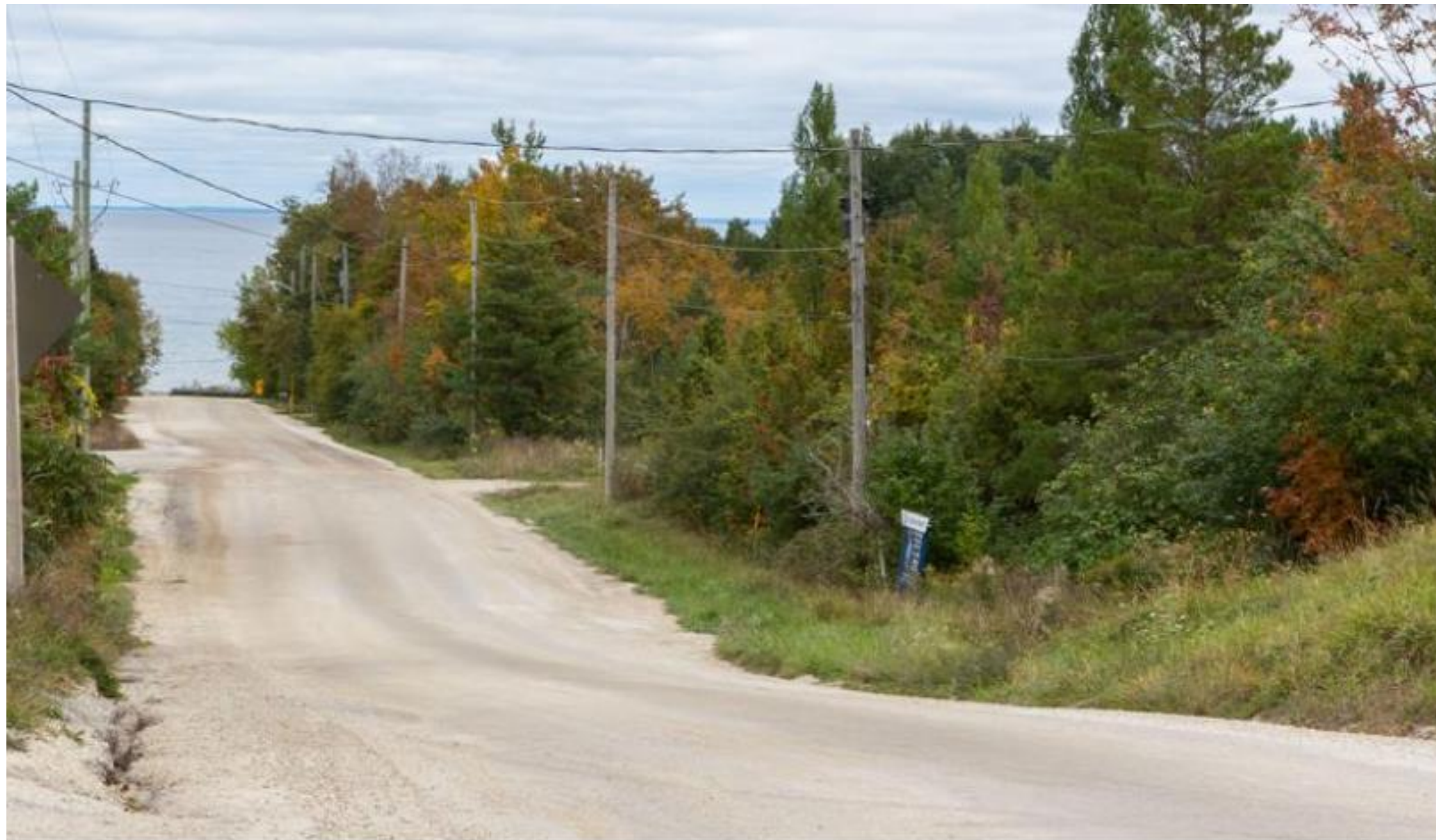
Peel Street North Road Reconstruction
