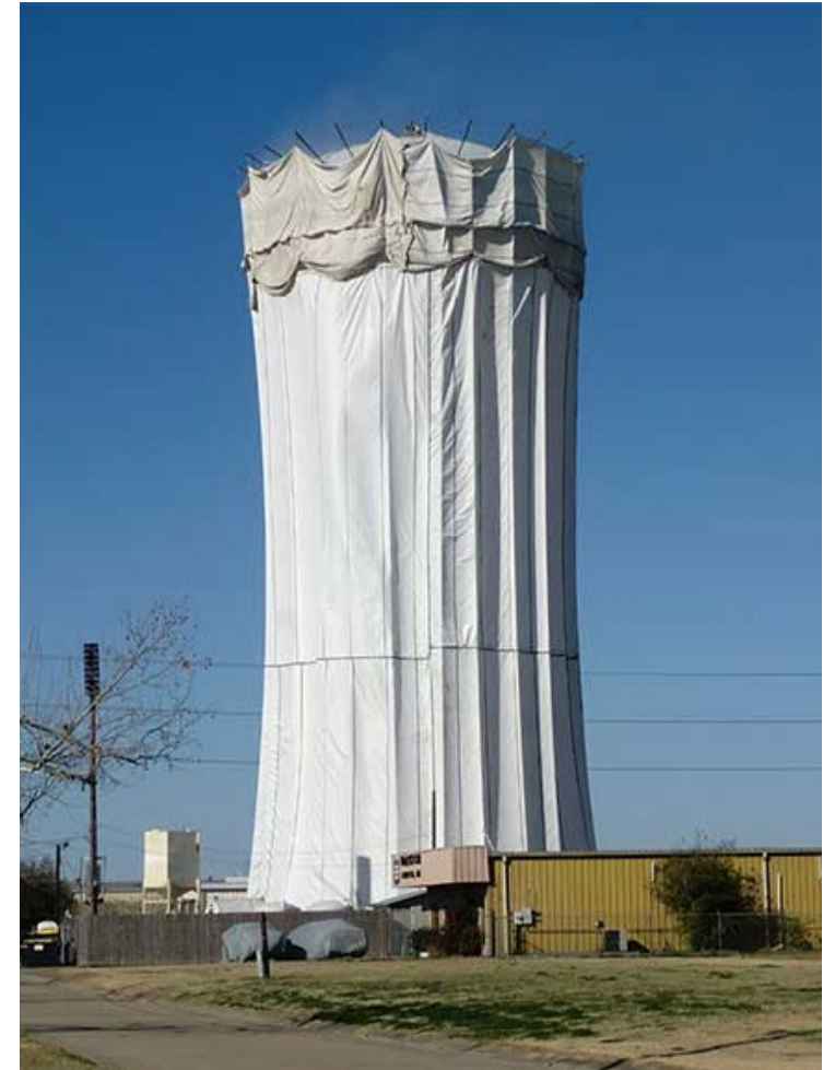
Image of Water Tower with lead containment shroud
