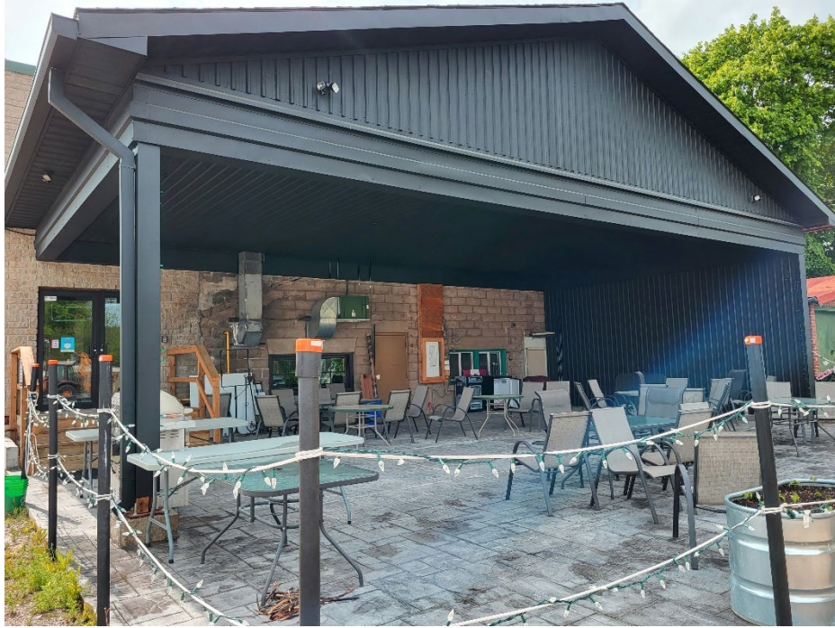
Marsh Street Centre patio project
