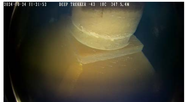
View down at roof support pillar to floor interface
