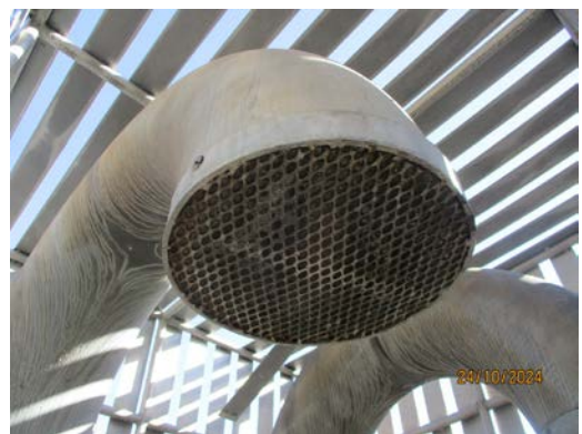
Vent two of two, screening is ok
