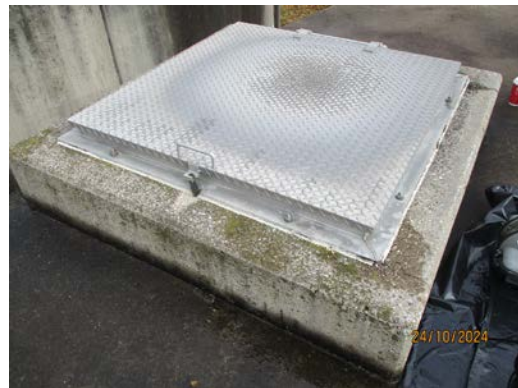
Roof hatch secured and locked after inspection
