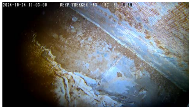
Floor to wall area; sediment cleared away by ROV
