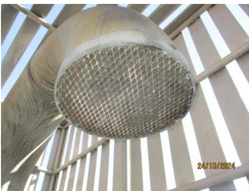
Vent one of two, screening is ok
