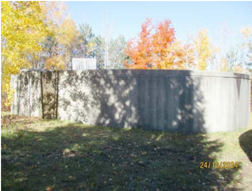
Overall view of the North Reservoir
