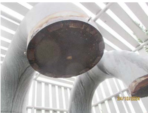
Underside of 1 st gooseneck vent screen – ok
