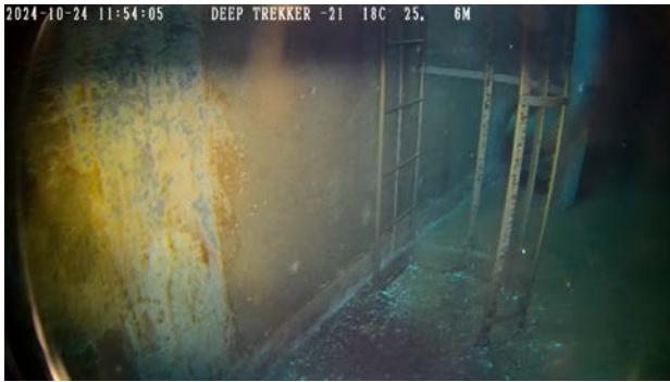
Ladder bottom, see pipe and support behind it
